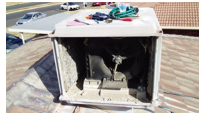
Evaporative cooler showing no maintenance.
