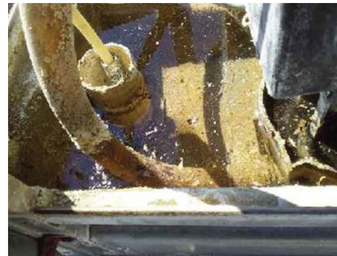
Lack of maintenance shows calcium build-up in sump of cooler.
