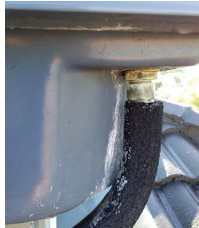
Poor maintenance shows water leaking from inlet valve.
