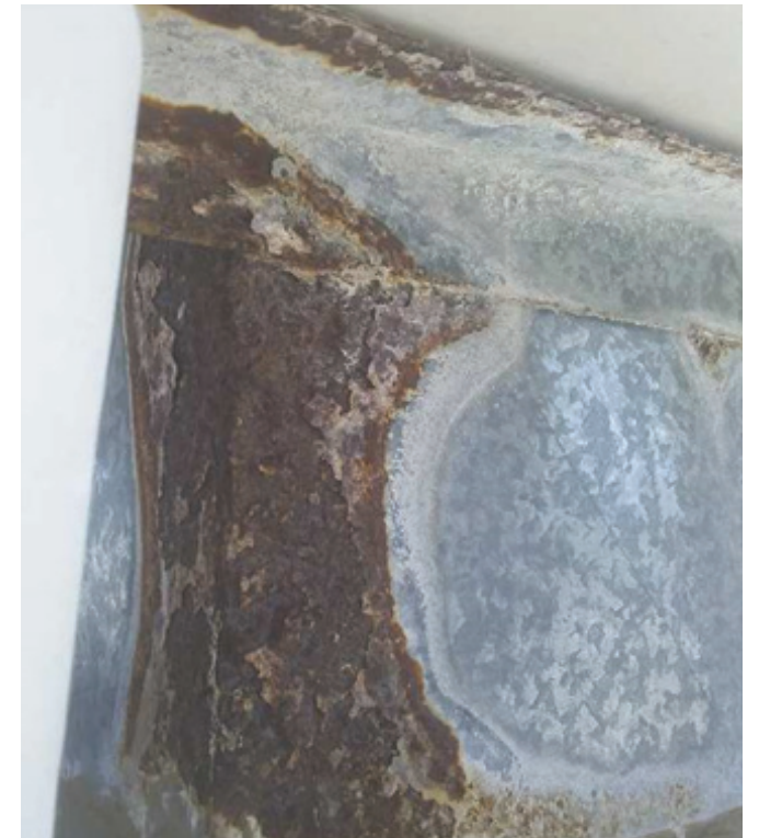
Water leaks on dropper causing corrosion.
