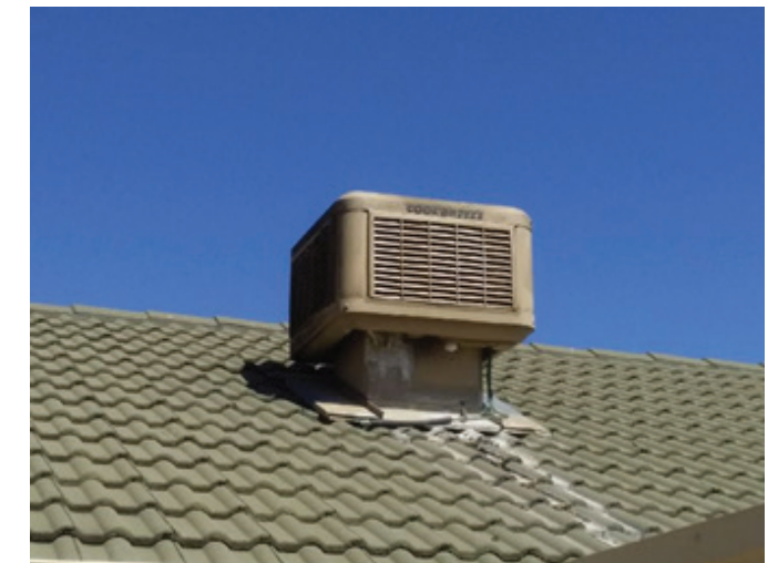
Evidence of water leaks with calcium stains showing on the tiles.
