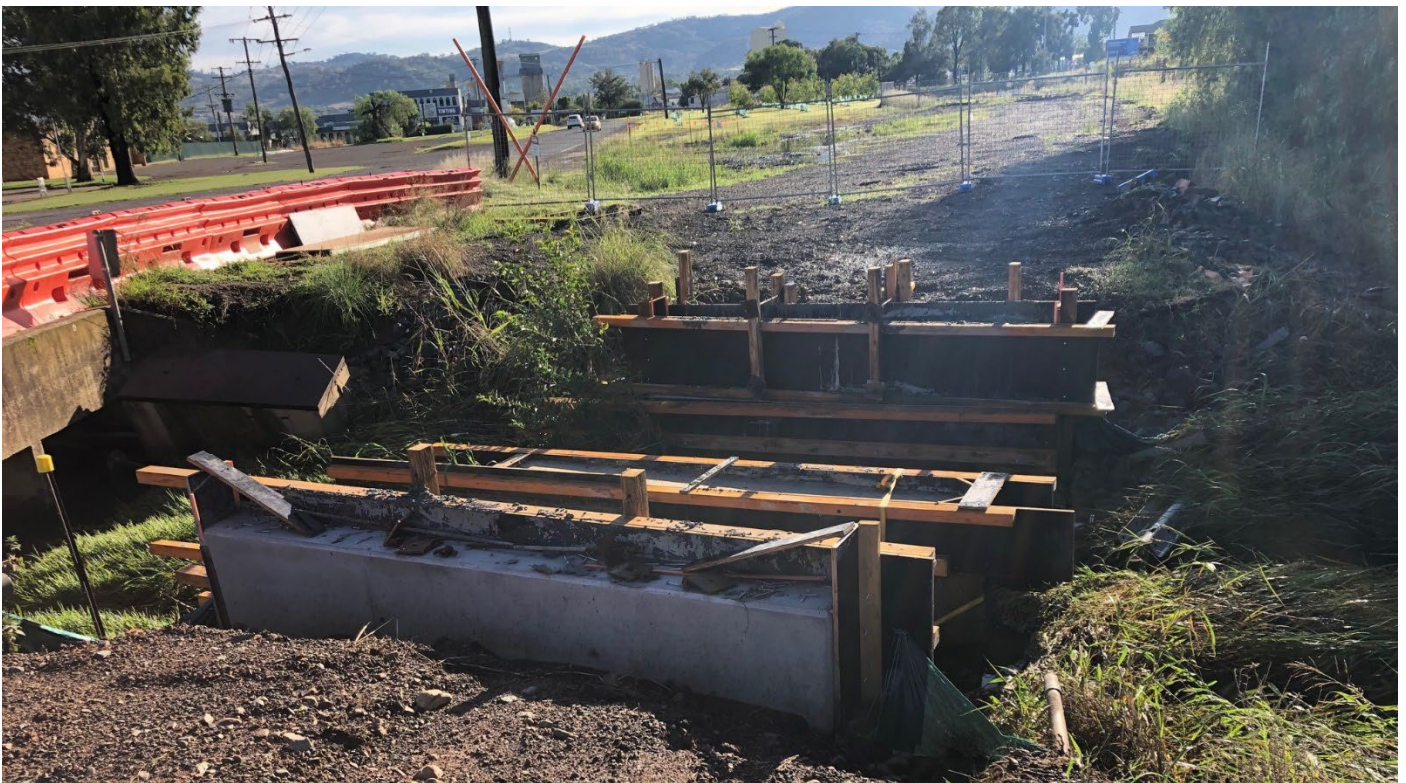
Image: Works continued on refurbishing concrete bridge piers during March. The bridge pictured is located adjacent to old Gunnedah Road and will have a new steel structure installed in April.
