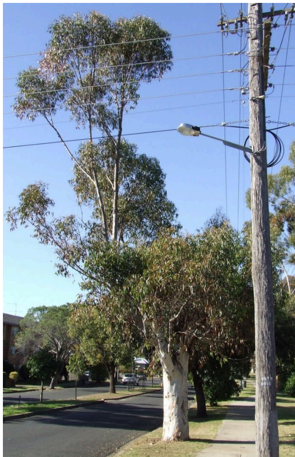
Tree limb impacting an overhead powerline in Gipps Street, Tamworth
