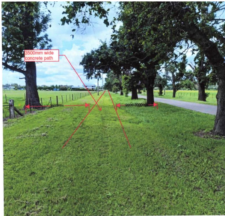
(Fig 6) Option 1: Between existing power poles and trees: Involves the construction of a concrete path approximately 500mm offset from the line of the power poles, leaving 2-3m offset to the tree line.
