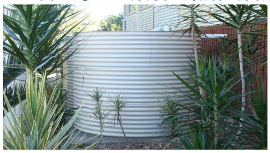
Rainwater tanks can be connected to the toilet and laundry of a home. This helps to maximise the benefits from the rainwater tanks as water can be used year around and not just during the dry months of the year.
